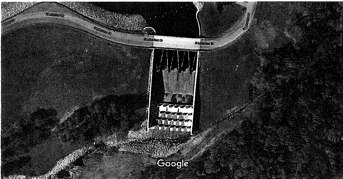
Figure 7 – Aerial View of the Lake Holiday Dam and Spillway
