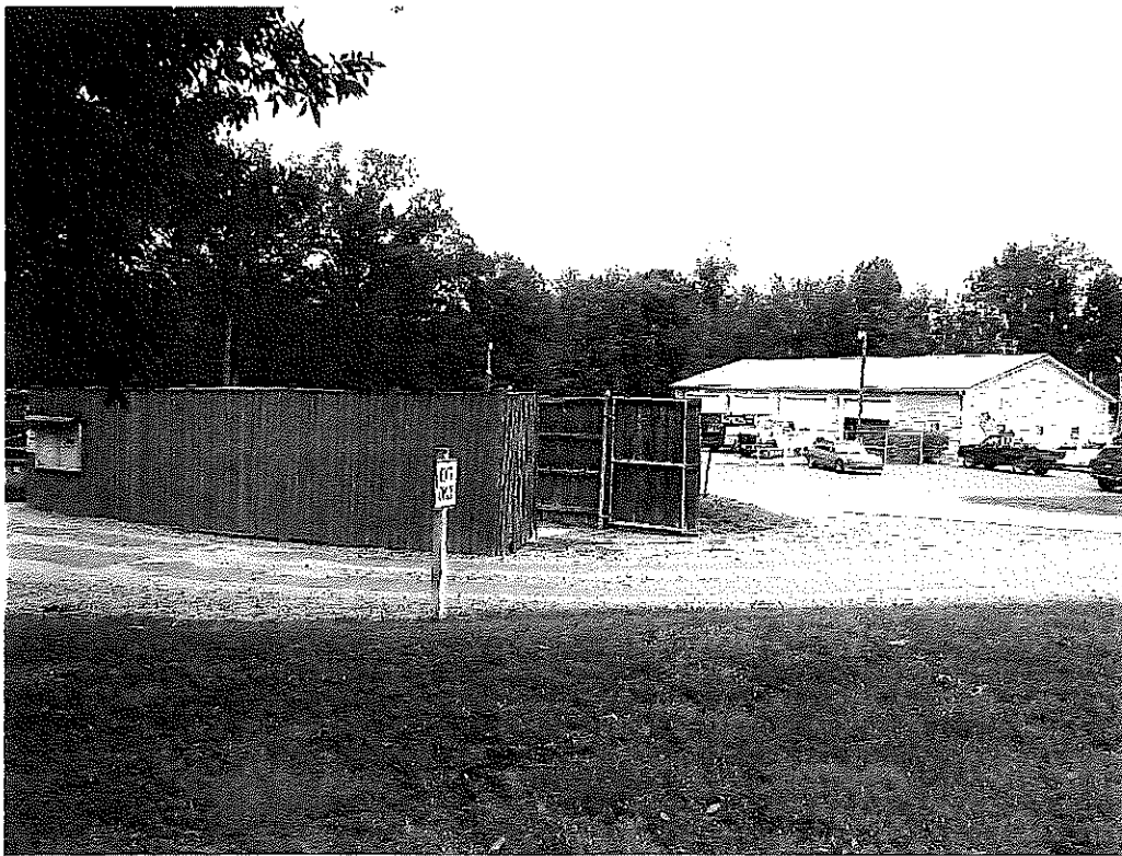
Figure 29 – Maintenance Building and Trash Facility
