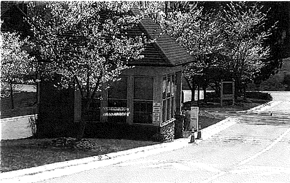
Figure 10 – Front Entrance Gatehouse
